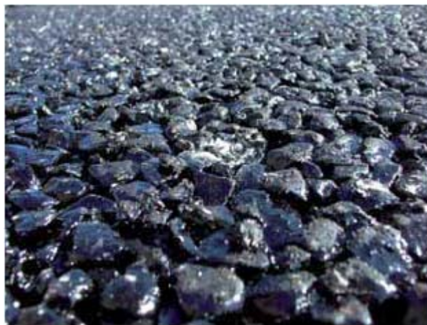
Porous asphalt from Lyngbyvej in Copenhagen
